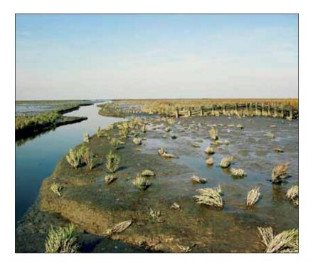
up and three artificial creek systems were dug which were to have a role in the supply and discharge of seawater and sediment. The creeks were designed in a winding pattern to give them a natural appearance. Their initial width was between 5 and 10 m. The soil dug up was used to raise the dike behind the saltmarsh along the adjacent summer polder in case of an increased risk of flooding.
